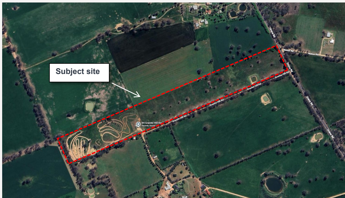
Figure 2 | Site Aerial (Google Maps 2026)
